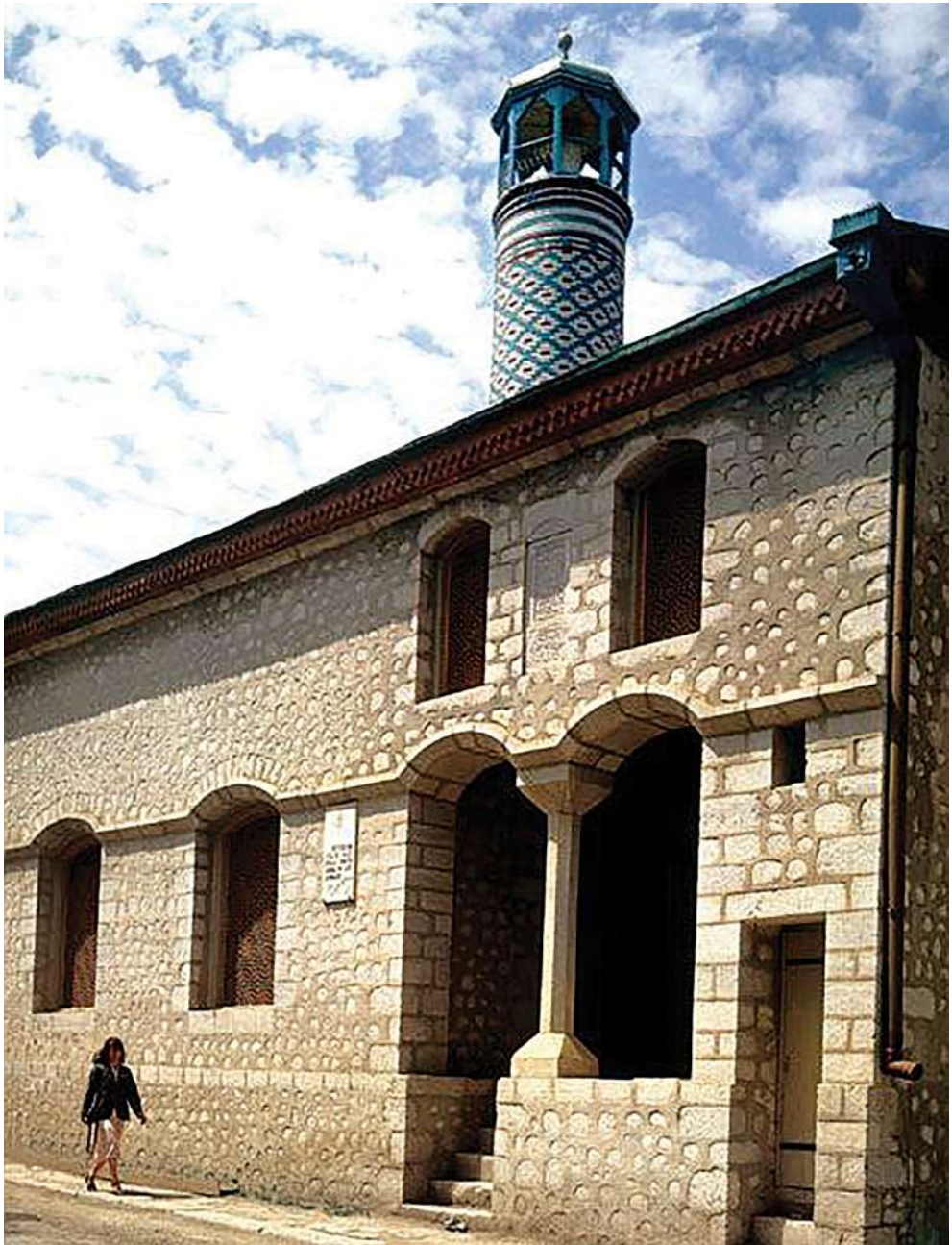
Fig. 3. Restoration of Saatli mosque.
