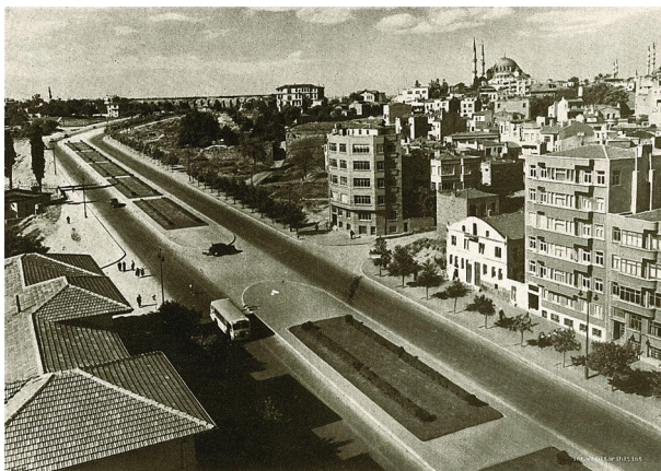
Fig. 4. Atatürk Boulevard view from Aksaray
