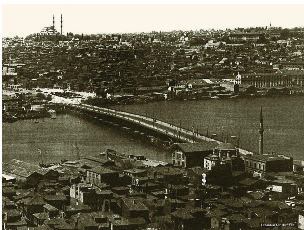
Fig. 3. Unkapanı bridge built over the Golden Horn
